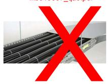
Metallic tray with cover to transport the cables and goes one cable to each room switch board.
